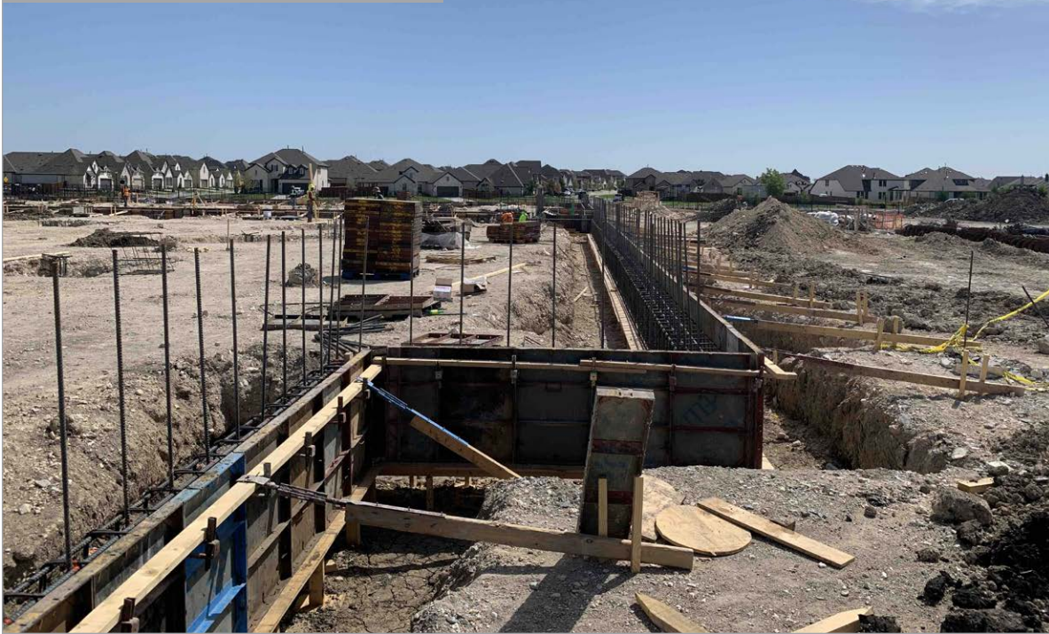
Grade Beam Formwork and Reinforcing
