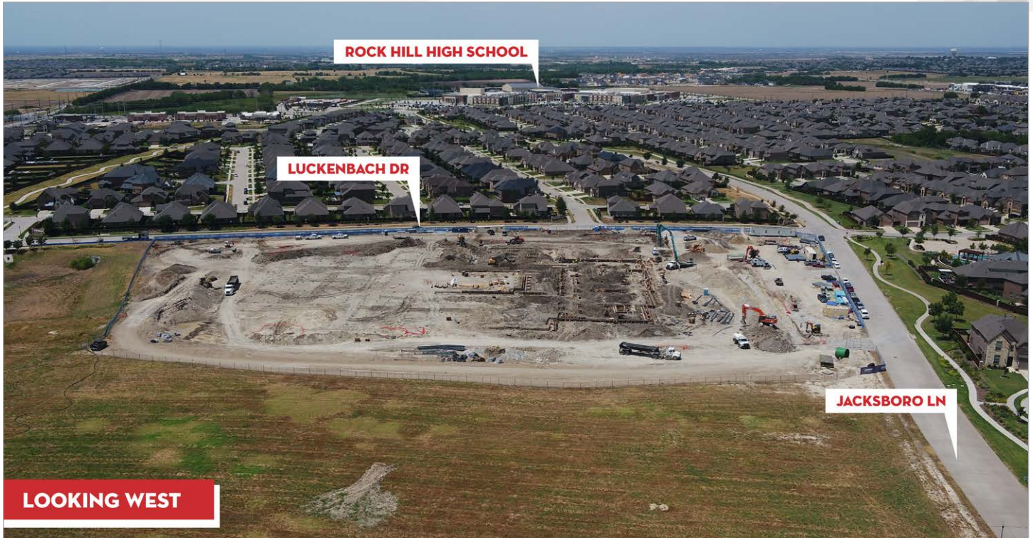
Underground Site Utility Trenching
