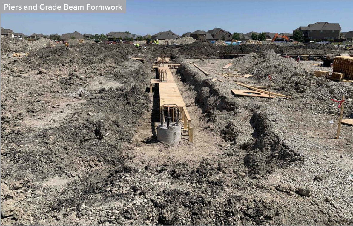
Grade Beam Formwork and Reinforcing
