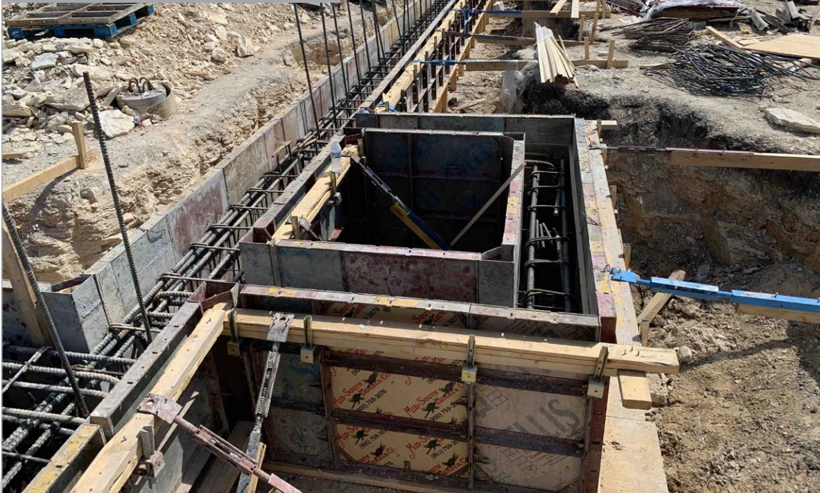
Grade Beam Formwork and Reinforcing
